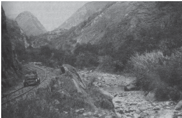
Figure 2. Railway construction at base of the Devil's Nose switchbacks, Ecuador, showing railway on the left and stone-lined riverbed on the right, where several pools can be seen (likely formed by falling rocks from construction), which would likely have provided suitable habitat for Anopheles pseudopunctipennis larvae. Photograph: Historical Archive of Banco Central and García Idrovo (14).
